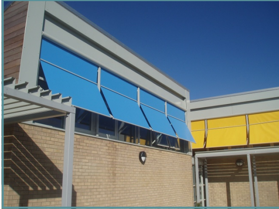
Blinds almost fully deployed
